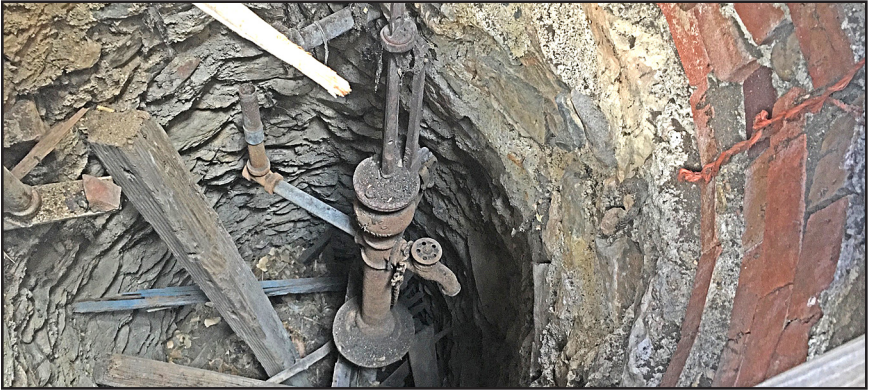
The brick encased subterranean well and pump piping below the ground of the lowest floor. – Photo © 2021 by Keith Sorci.
