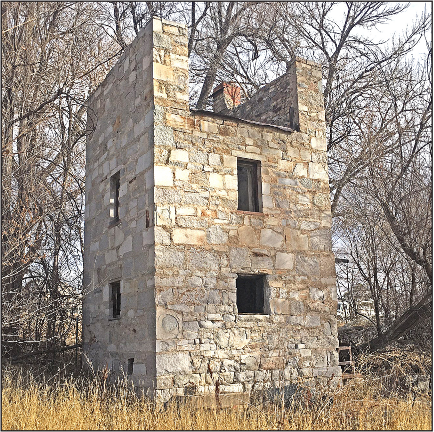
The 14-foot square, three story building constructed of rare granite and marble from the Glencoe Quarry, a quarry that is now under Ralston Reservoir. – Photo © 2021 by Keith Sorci.
